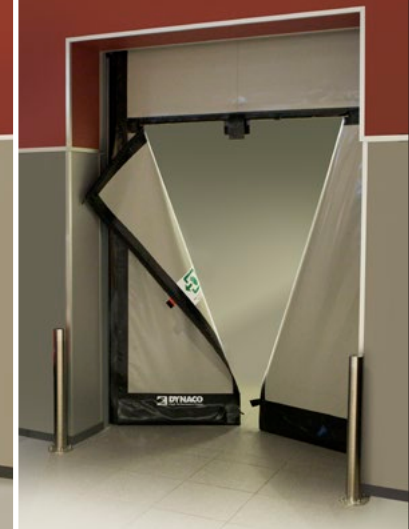
Emergency exit open
